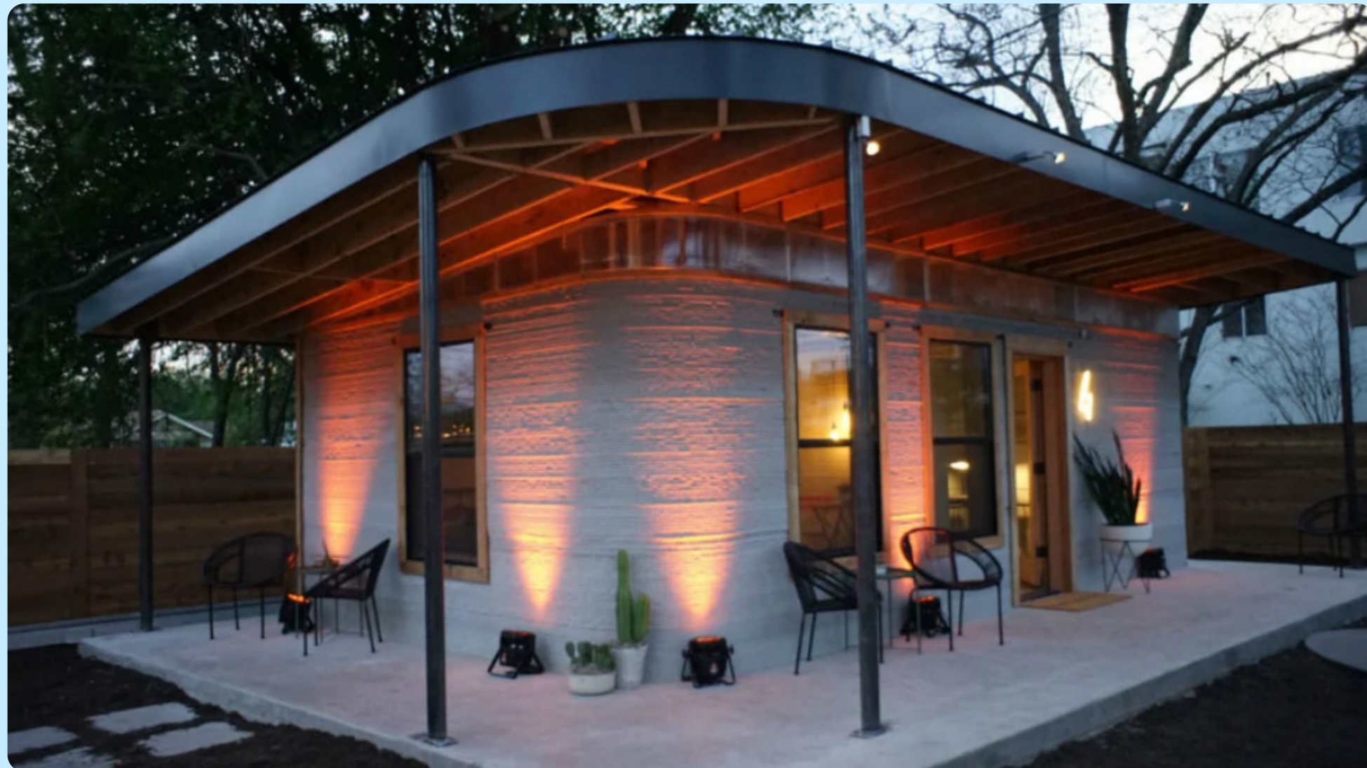
A 3D printed house. Source: Singularity Hub
